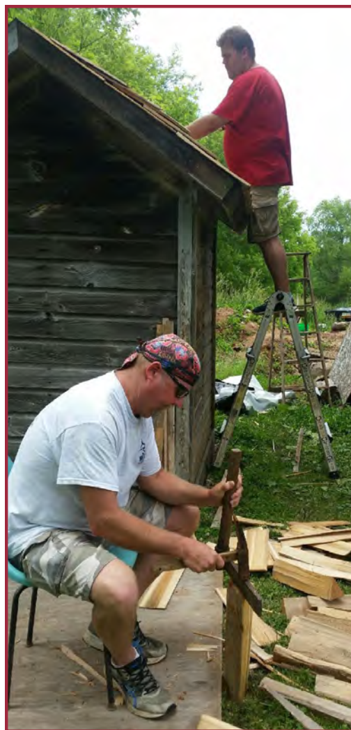
Nath Chisholm (on ladder) attaches a newly split cedar shake.
