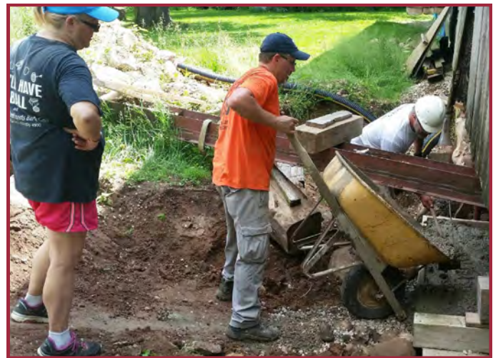
Julie & Tim Chisholm mix and pour cement for the footing under the northwest corner of the Housebarn 1870's addition on June 17.
