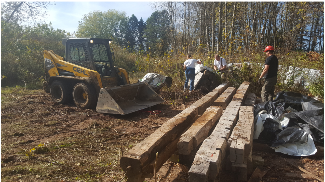
Over the years, replacement timbers were collected and recycled into the timber framed Housebarn. There are no nails in the timbers, they are held together with pins (tenons) and square holes (mortises). Many buildings were able to be moved or reconfigured as farms expanded and adapted to new trends in livestock and cropping.
