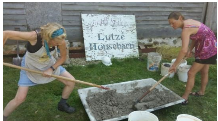
Kathy & Amy are manual mortar mixing on a 90 degree workday
