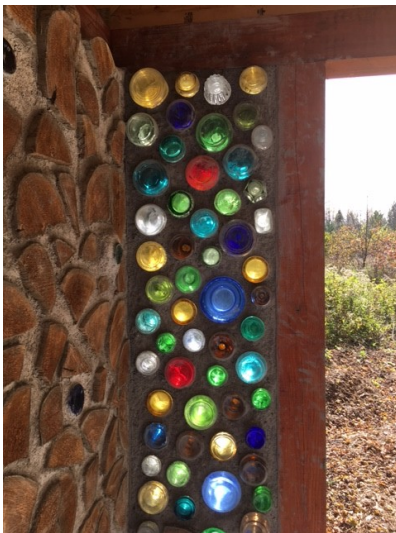
Close Up of bottles embedded in the mortared wall to bring ambient light into the new structure
