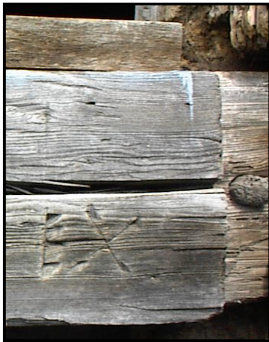
Numbering system for the logs as to where they should be placed.
