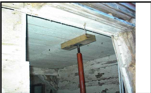
The entire Housebarn had jacks placed so nothing would shift or collapse as work was done.
