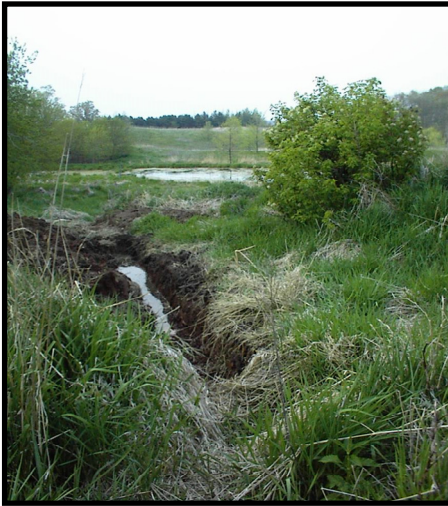
Drainage from the floor in the fruit cellar was led out through a wooden drain pipe. That drain outlet is on the side of the north hill, here you see extra perimeter drainage outlet we added.
