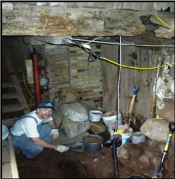
Above and below: The wall at the bottom of the fruit cellar stairs had collapsed and had to be replaced. Here Bob Faye does an exploratory dig.
