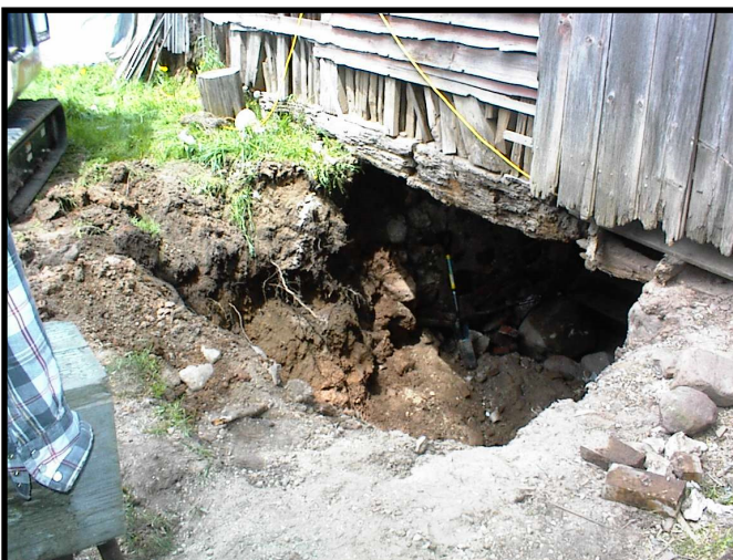
Above and below: The wall at the bottom of the fruit cellar stairs had collapsed and had to be replaced. Here Bob Faye does an exploratory dig.
