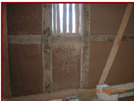
Completed nogged clay packed wall.
