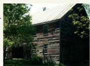
The rectangular structure, 72'-9" (east-west) × 28'-5" (north-south), was constructed with a hand-hewn, post and beam timber frame with clay "nogging"
