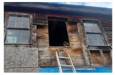
Installation of vertical & cross timbers where 1930's window has been removed in the 'chicken coop' area ^^^
